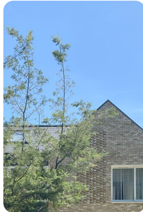
Figure 19 | Example of Brick Detailing, Fletcher Crane Architects
