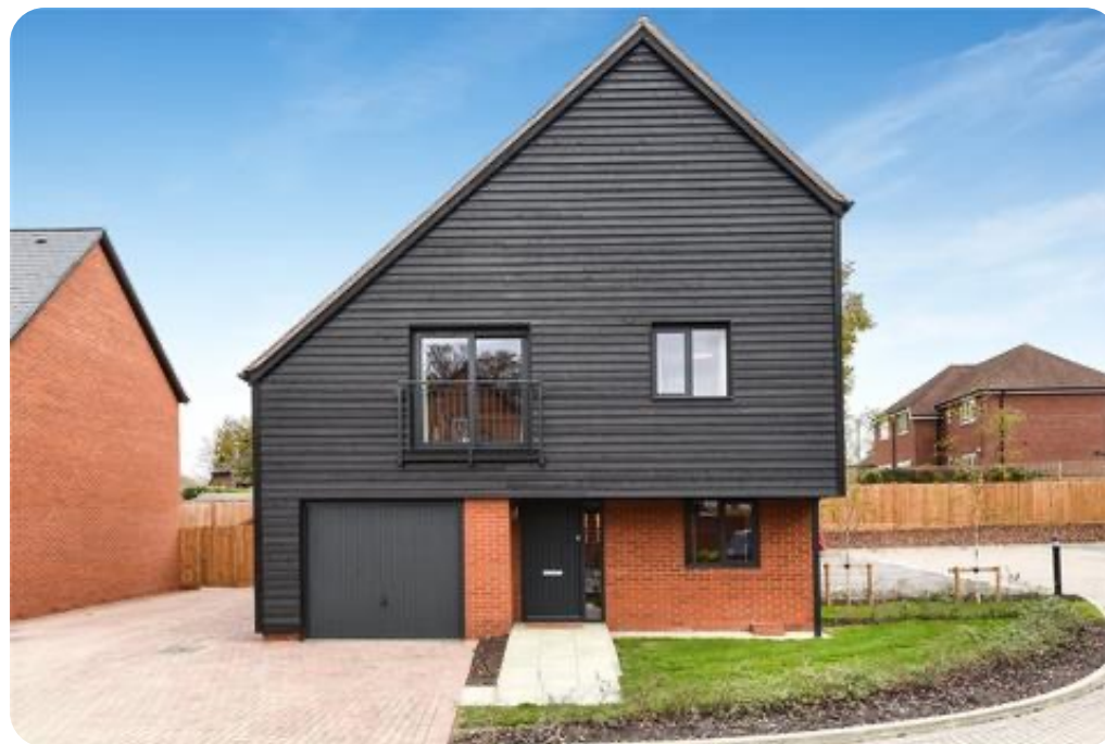
Figure 23 | Example of Material Finishes, Station Drive by Snug Architects
